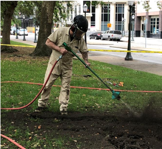
Radial Trenching in Mobile. AL
