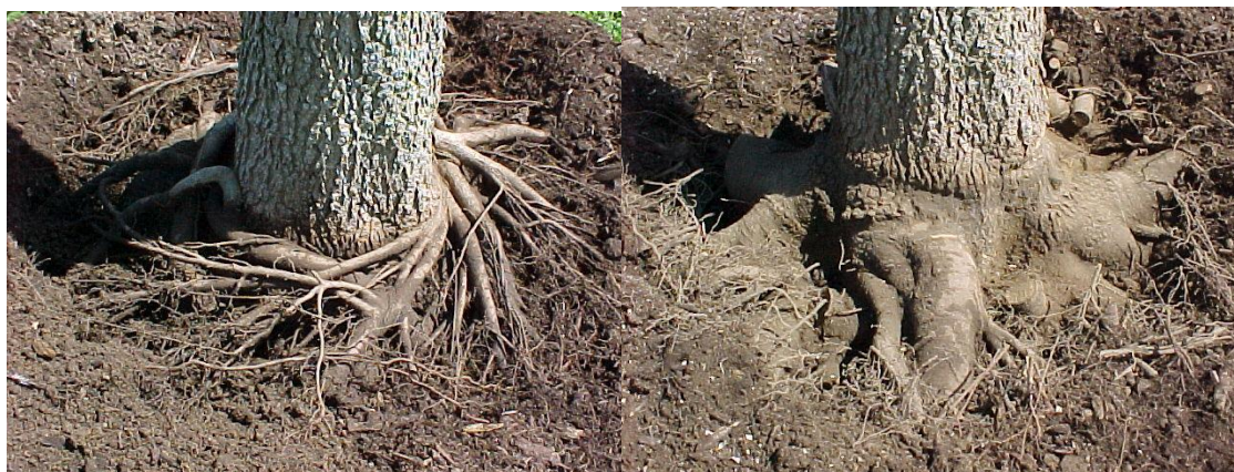
Root Collar Excavation Before and After
