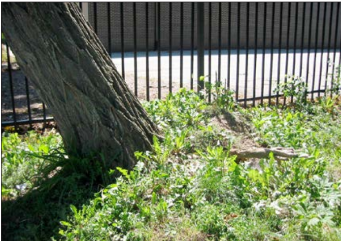
Root failure often leaves trees leaning. Look for exposed roots after high wind storms.
